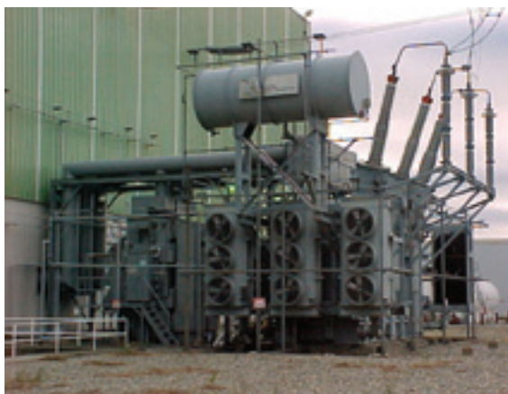
Figure 1: 650 MVA GSU
