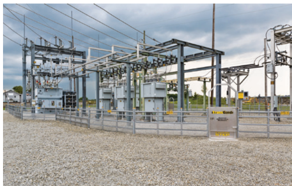
Complete installation: patented, modular design delivers mild electric shock preventing climbing animals from entering the facility
